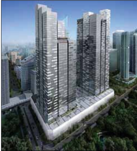
The towers are over 220 metres high and were presented with the coveted Green Mark Platinum Award
