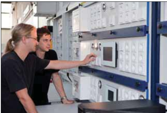
The touch screens on the test stands indicate whether the load management functions are as required
